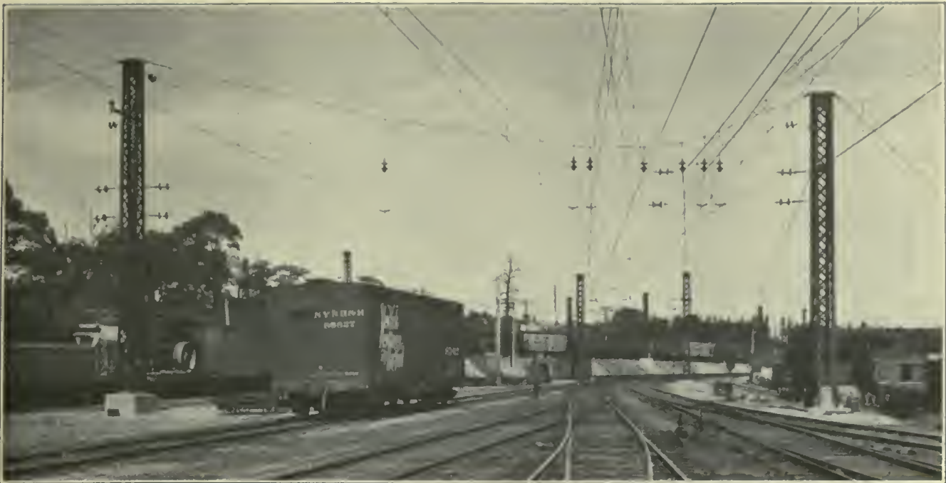
FIG. 519. OVERHEAD CONTACT SYSTEMS. Yard Track Construction. 11,000-Volt Single-Phase Electrification South Norwalk Yard, New York, New Haven & Hartford Railroad.
